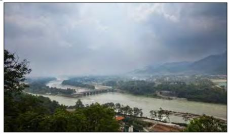
repeatedly heating and cooling the rock to crack and weaken it. The system also includes a dike in the middle of the river to help reduce the amount of silt that flows into the aqueduct. A spillway allows excess water to continue down the Minjiang River to prevent the flooding of the Chengdu basin. The Dujiangyan Irrigation System is a pearl in the water works construction of ancient China. Built over 2,200 years ago, it still provides benefits for the people.
